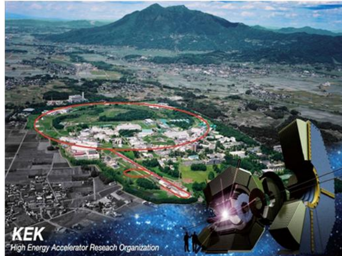
Figure 2.3: Aerial photograph of the KEK laboratory
